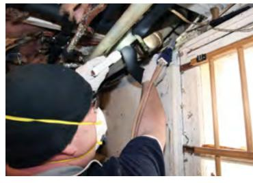
Advantage Weatherization worker seals air leaks in a basement to help stop drafts. ©2012 Advantage Weatherization, Inc.
